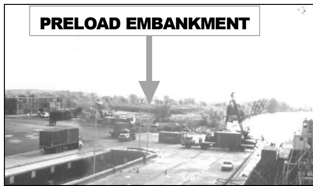
Figure 2. Preload embankment as seen from the wharf.
